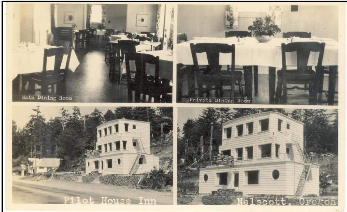
Figure 26 – The modern metal awning at Nelscott’s Foon Hing Yuen building (see here c.1946 as Pilot House Inn) presents another mural opportunity. From the Collections of the North Lincoln County Historical Museum and Society, Lincoln City, Oregon.
