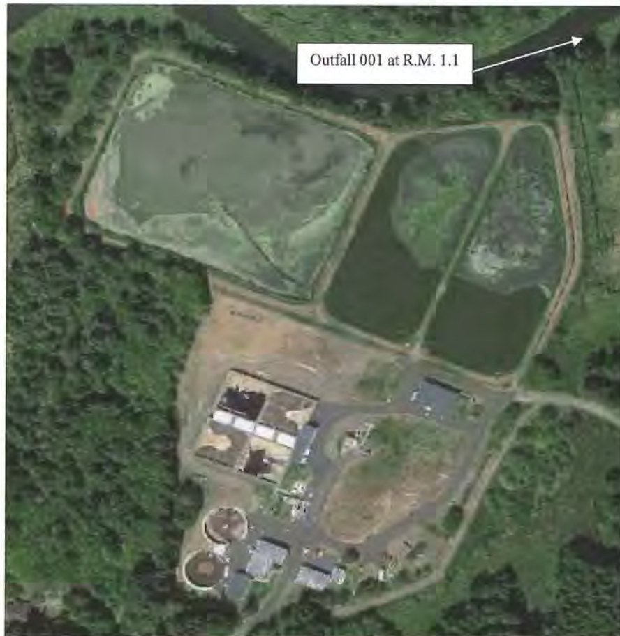
Figure 1: Lincoln City Wastewater Facility
