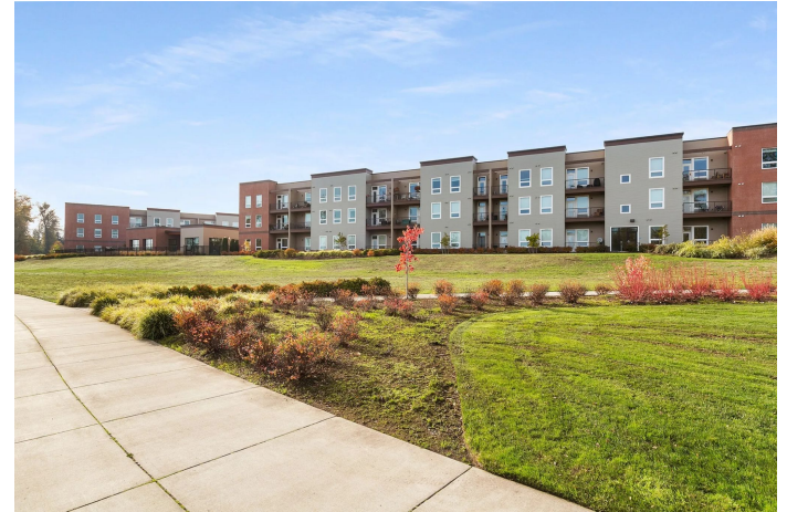
The City of Lincoln City invested in streets and utilities to get the Lincoln City Landing site "shovel-ready" for housing development.
