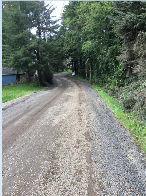
SW Bard Road Local Improvement District (LID)
