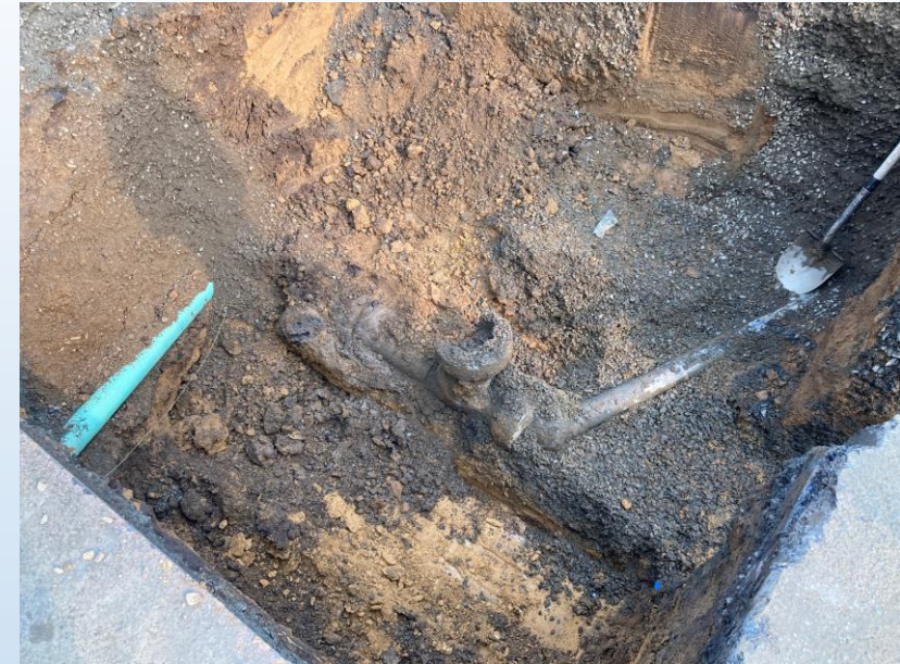
Degraded Sewer “Lamp Post” Replaced
