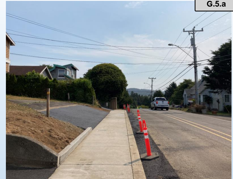
Narrowed Driveway & Slope Change
