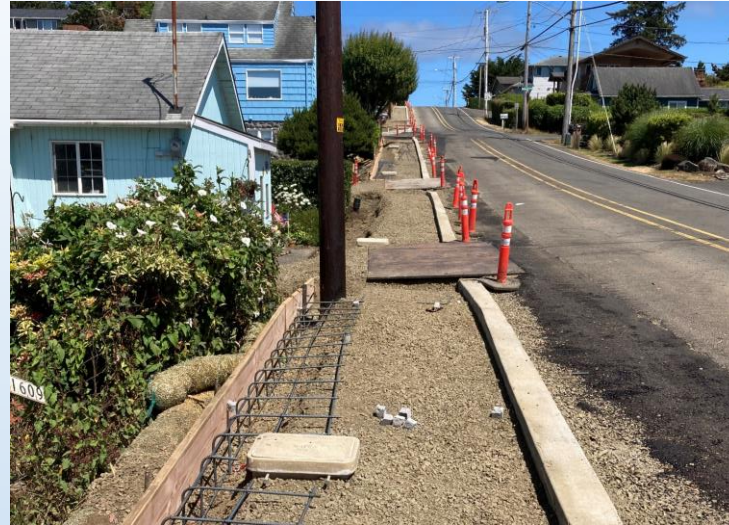
Exactly 4 feet – the minimum clearance in front of power pole.
