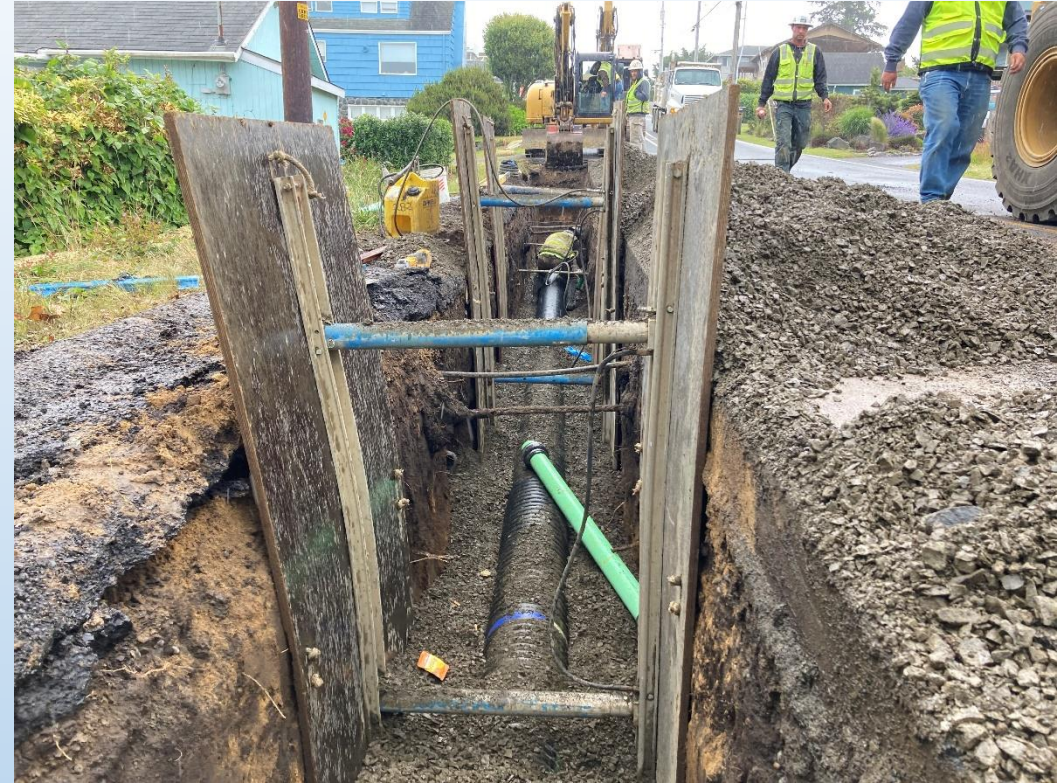
Storm Main Installation
