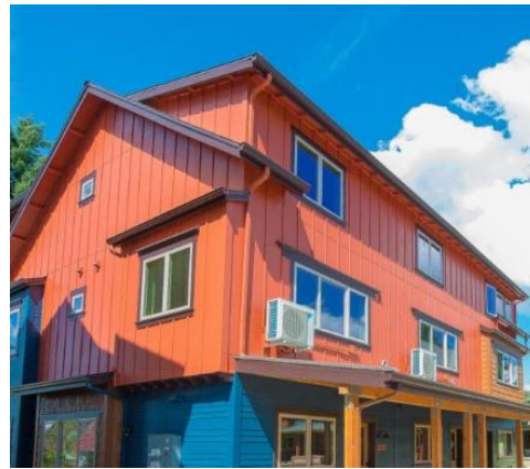
Pitched roof with attached shed roof.
