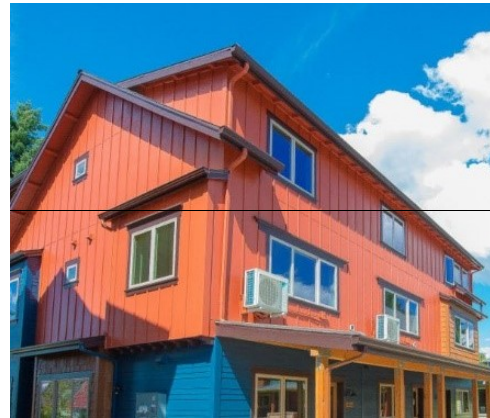
Pitched roof with attached shed roof.
