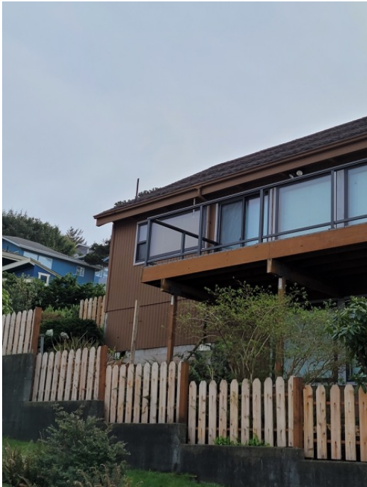
View from north side post-repair—March 1, 2021
