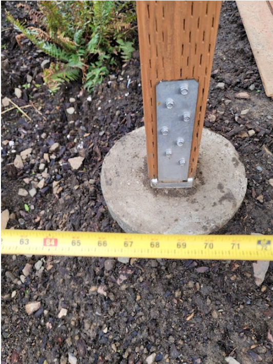
Set back of vertical footings north side—March 1, 2021
