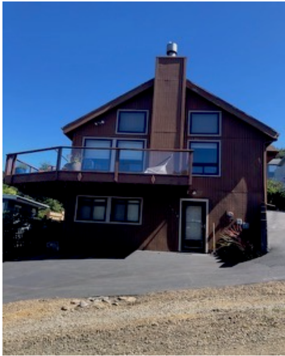
View from west side pre-repair—circa June 2020
